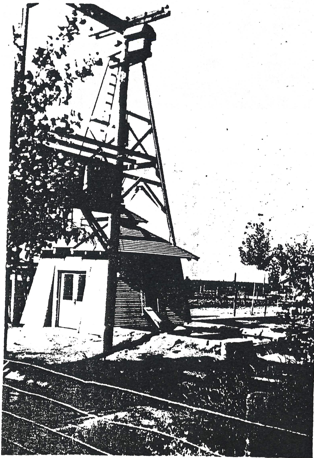
An electric pumping installation ca. 1920. (Phoenix Public Library)
