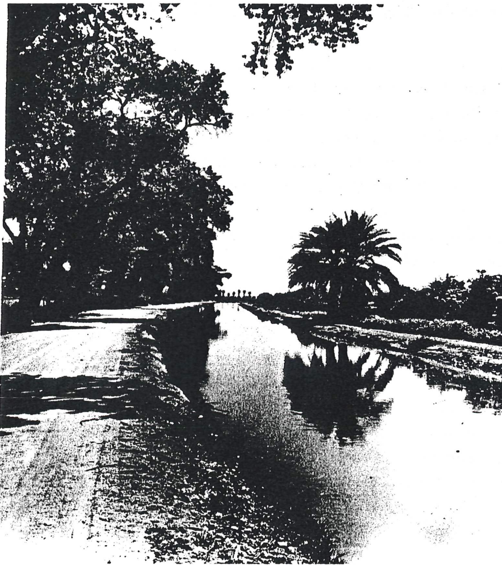
Western Canal before concrete lining. (S.R.P. Archives Collection)
